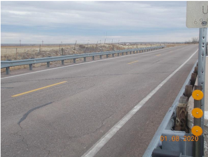
View of bridge M-22-U looking north.
